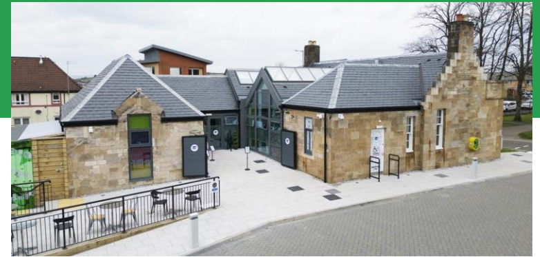
Cowan Park's gate lodge has been transformed.
