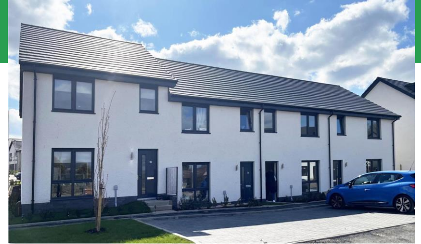
New council houses in Maidenhill will be delivered.
