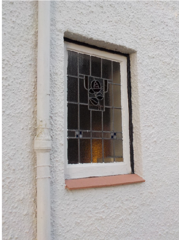
Photograph No.15 – Typical window detail
