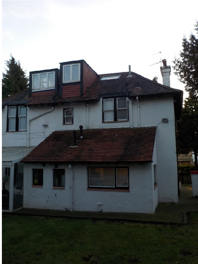
Photograph No.9 – Rear elevation
