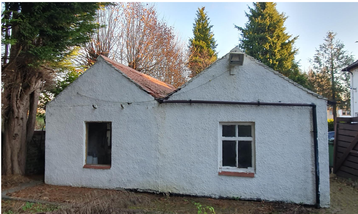
Plate 6. Garage from northwest (rear)
