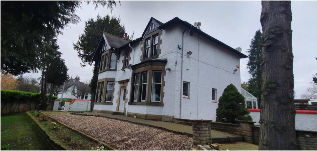
Plate 1. Front and north gable of building B1
