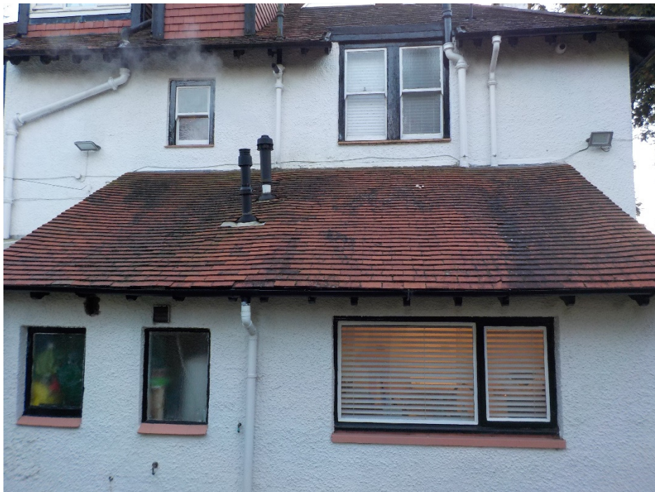
Photograph No.10 – Rear extension roof
