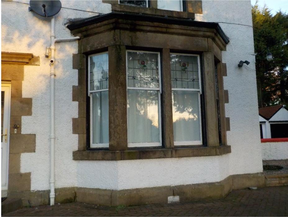
Photograph No.1 – Front right-hand, ground floor bay window
