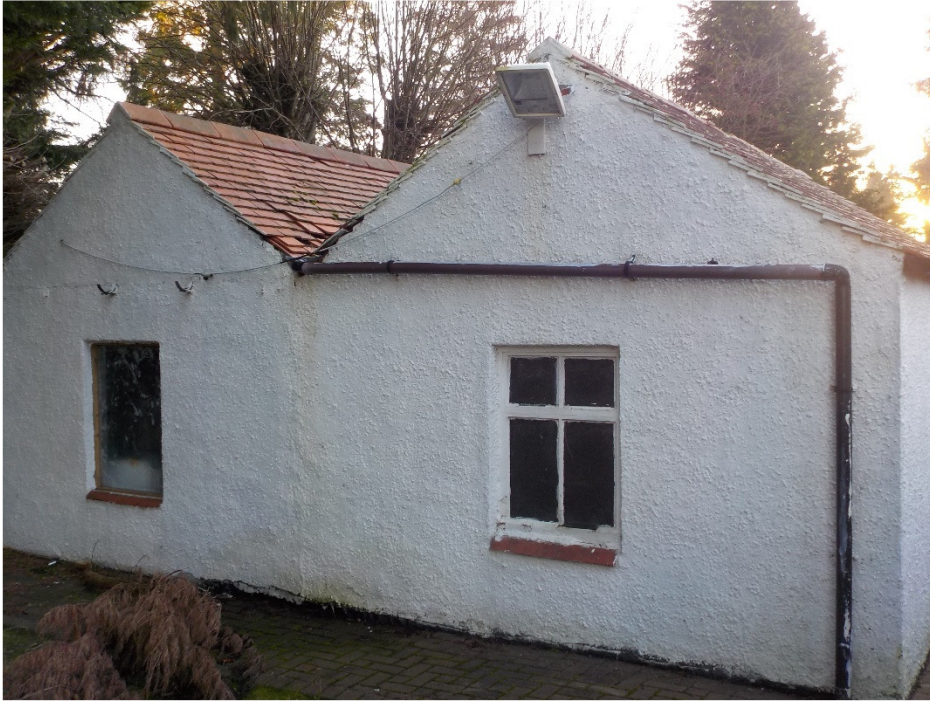
Photograph No.23 – Rear elevation of garage
