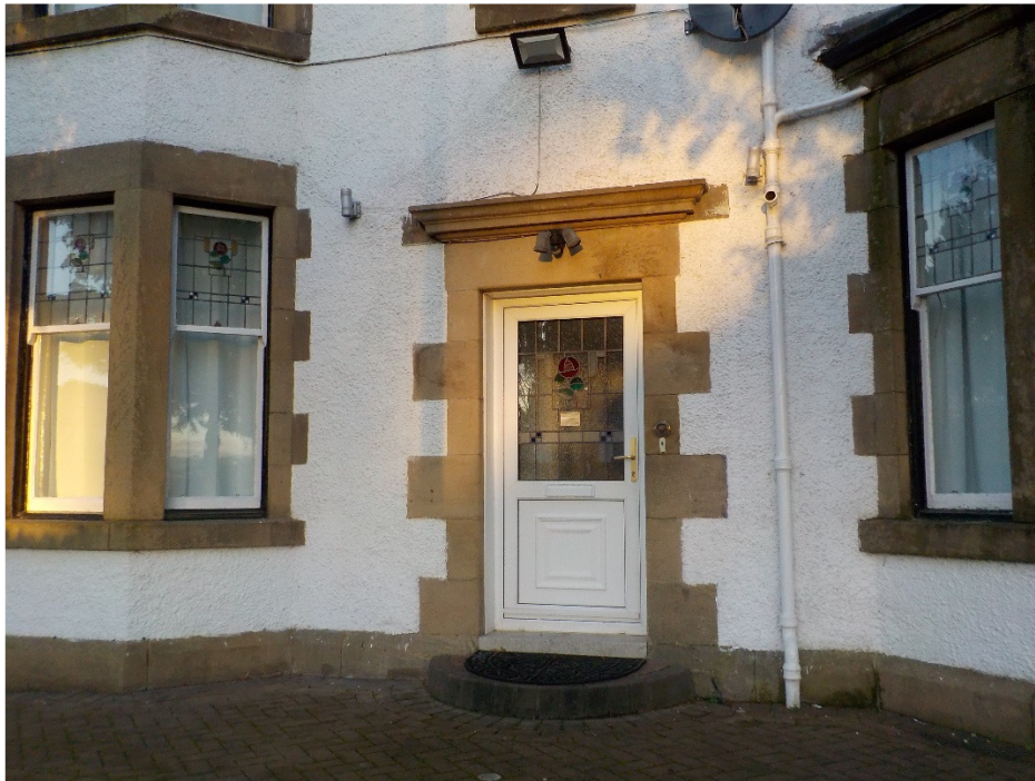
Photograph No.7 – Front entrance door
