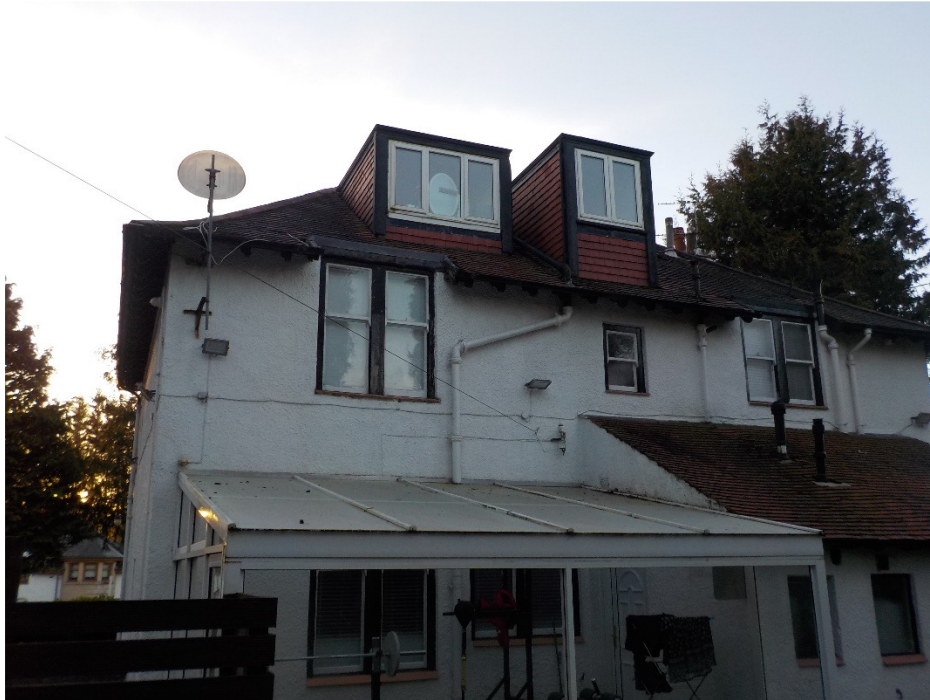
Photograph No.11 – Rear elevation
