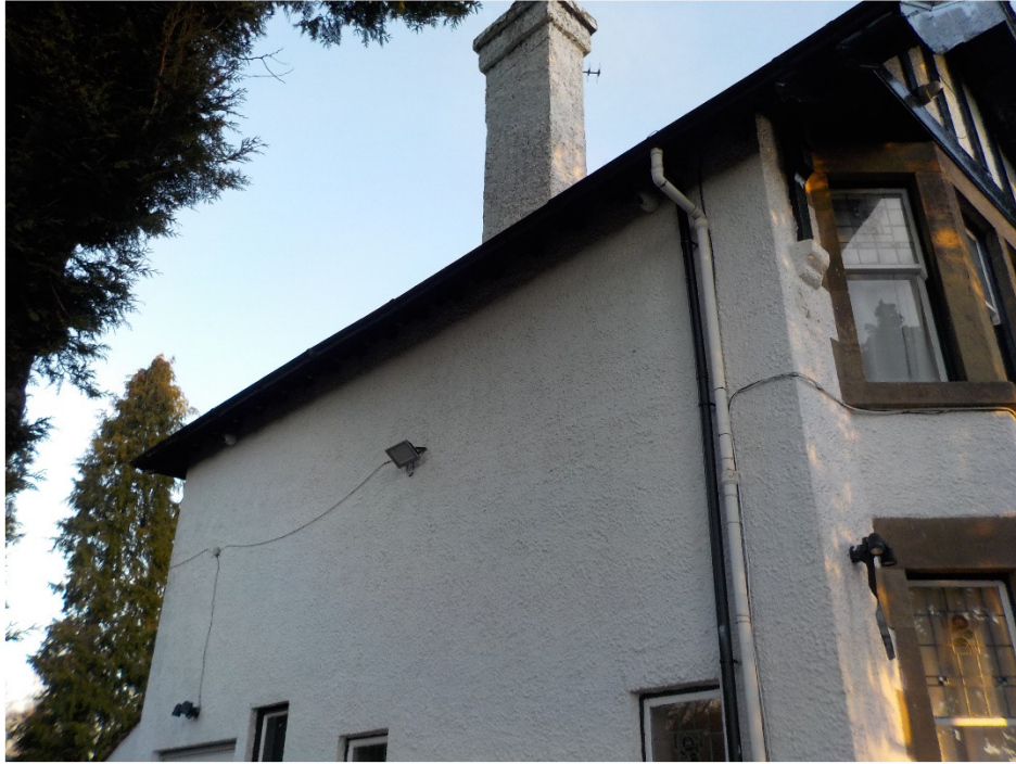
Photograph No.7 – Left-hand gable elevation
