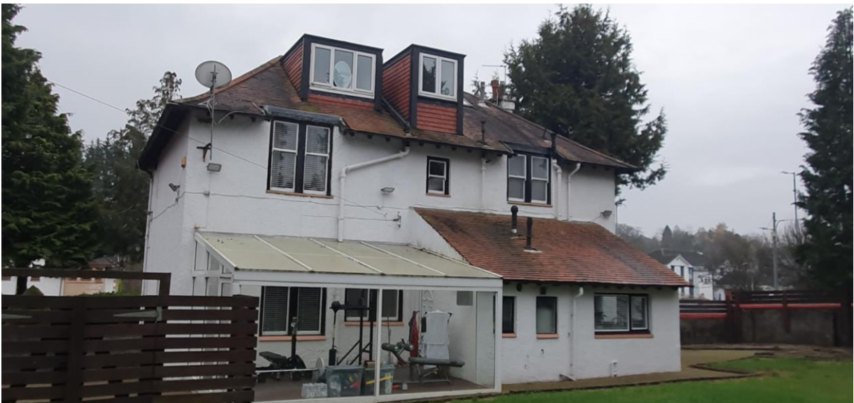
Plate 2. Rear of building B1
