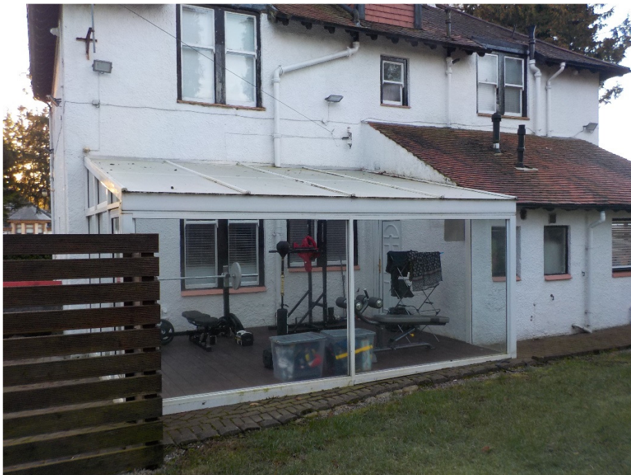
Photograph No.12 – Rear elevation
