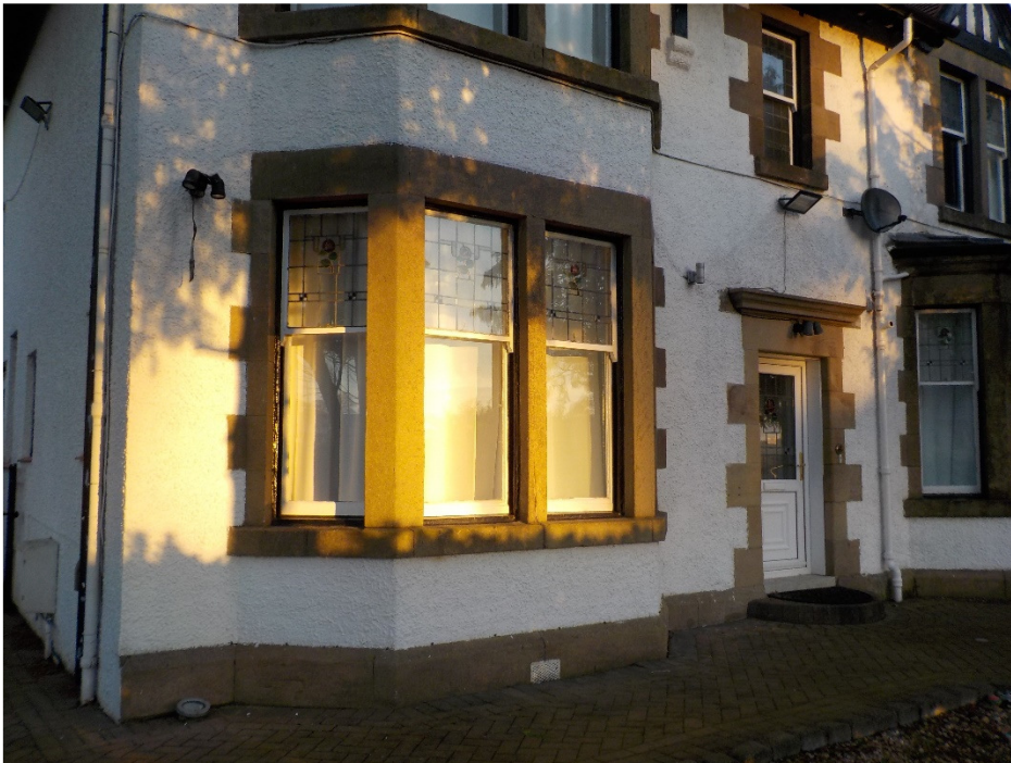
Photograph No.4 – Front left-hand, ground floor bay window
