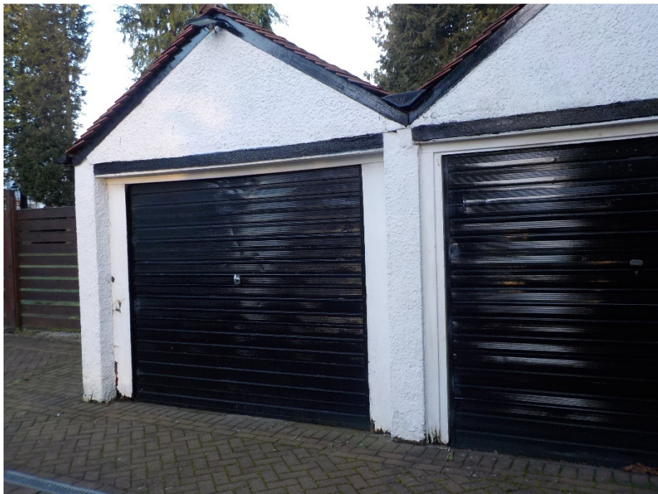
Photograph No.22 - Front elevation of garage
