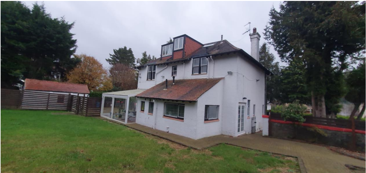
Plate 3. Rear of building B1 and south gable. Garages (building B2 in left rear)
