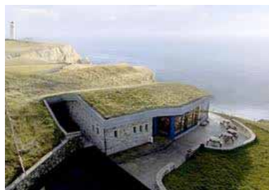
Green Roof, Stranraer
