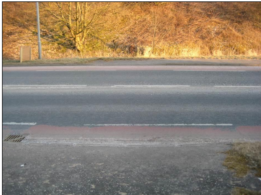
Existing dropped kerb crossing
