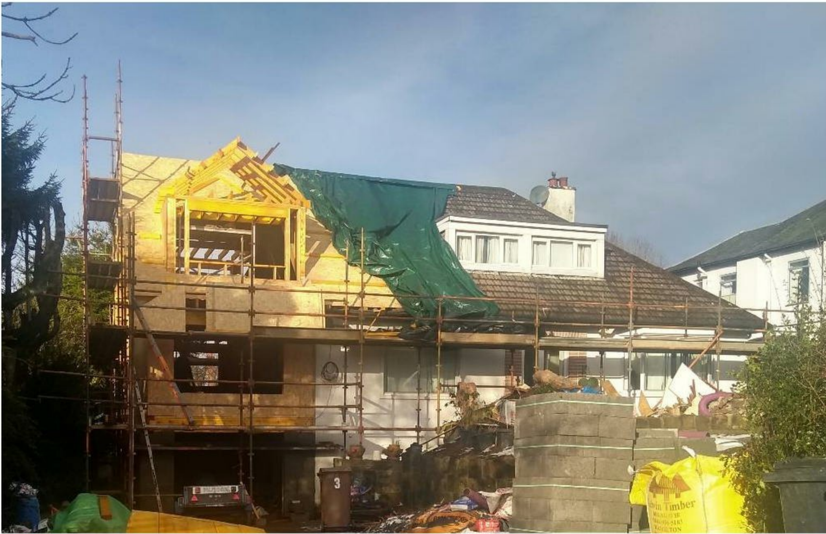
Image # 1: 3 Craigie Drive remodel in progress
