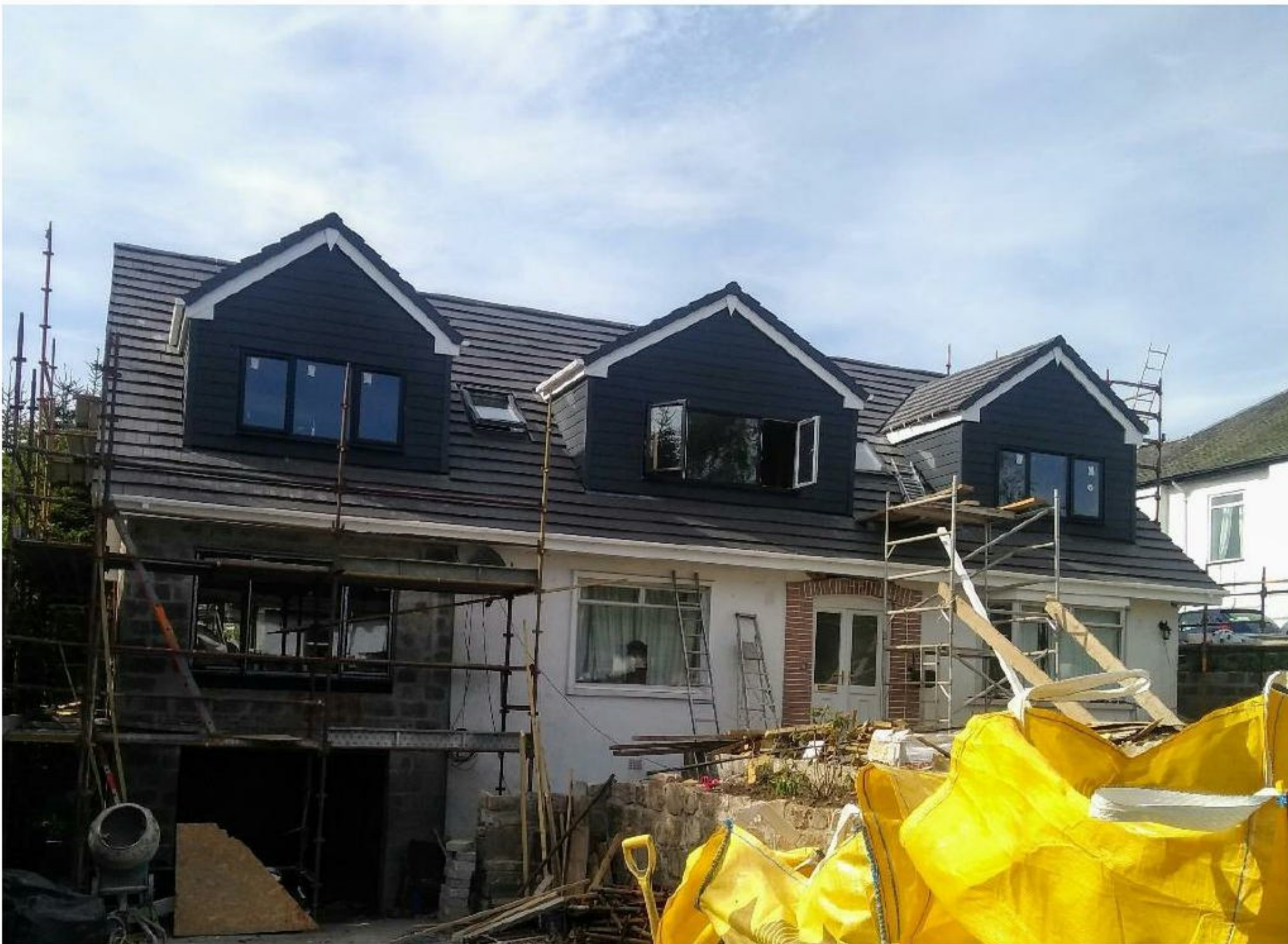
Image # 2: 3 Craigie Drive remodel nearing completion
