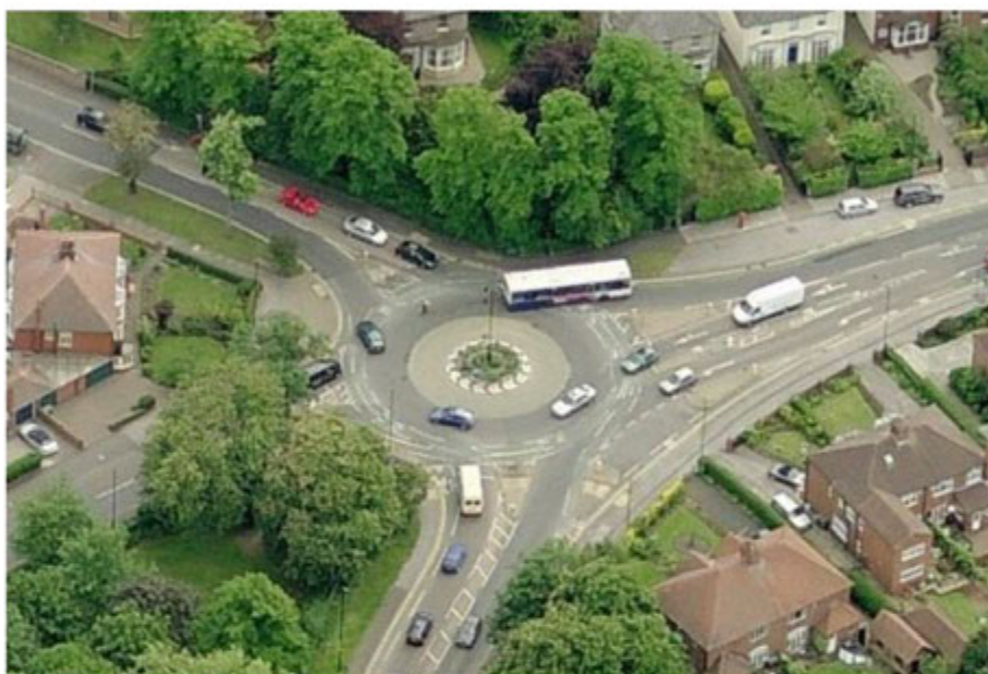
Figure 11 - Heworth Green Roundabout, York
