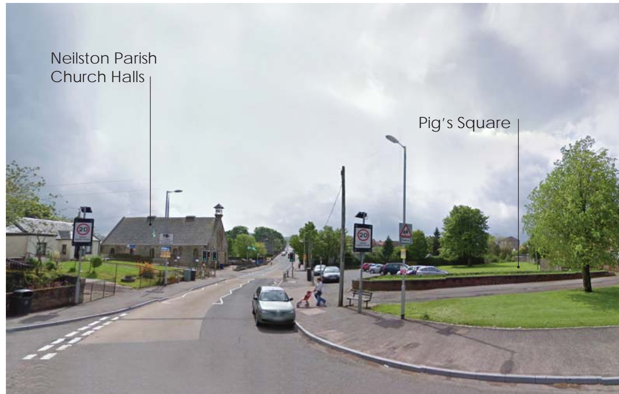
High Street looking south
