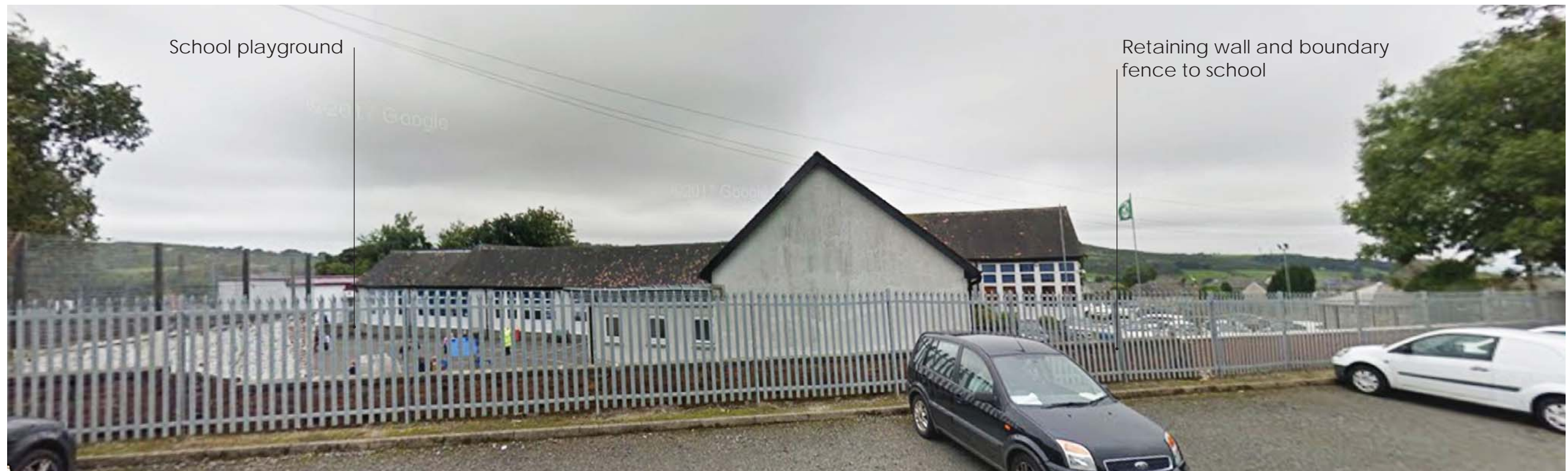
View from Broadlie Court car park looking north
