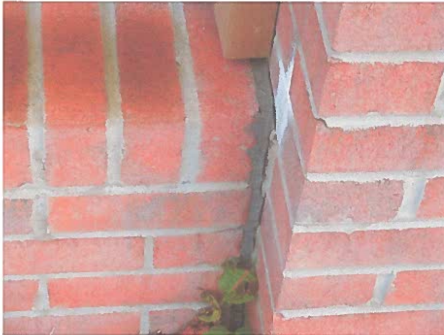
Internal View of Typical Movement Joint
