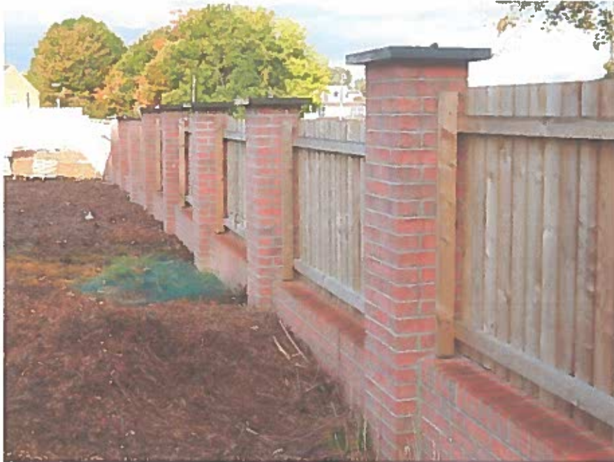
View on Inside Face of Wall Showing Nature of Construction
