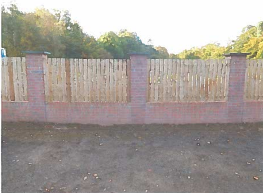
View on Outside Face of Wall Showing Nature of Construction
