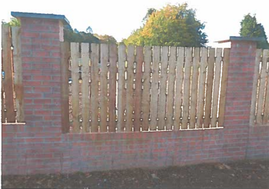
Outside View of Timber Infill Panel
