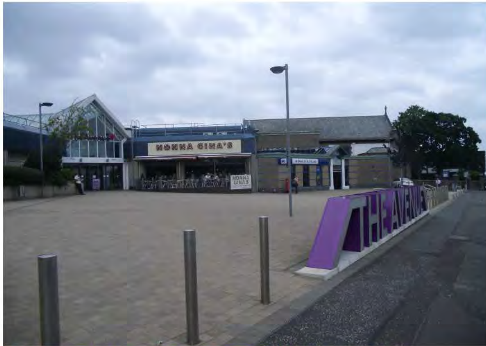
'THE AVENUE' SHOPPING CENTRE AFTER REGENERATION WORKS
