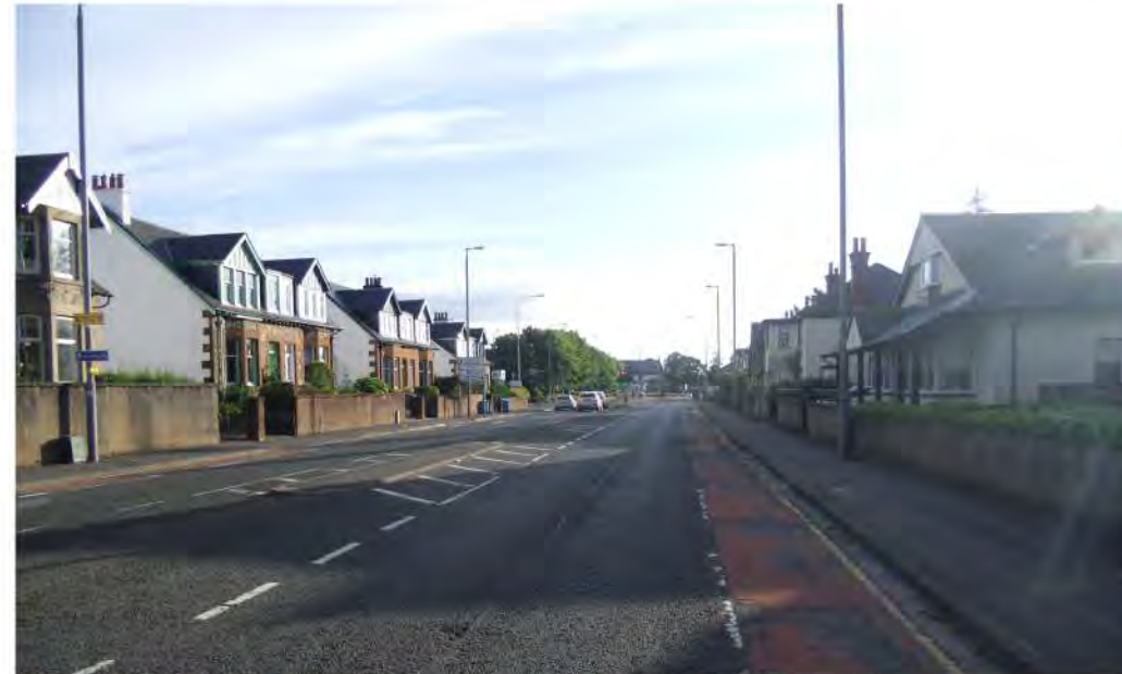
VIEW OF WESTERN APPROACH TOWARDS NEWTON MEARN'S TOWN CENTRE
