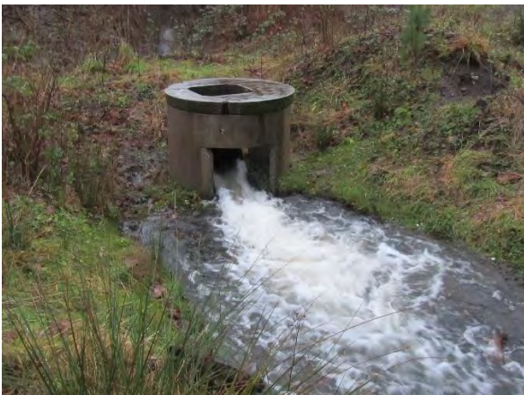
Figure 3 - Burn 'E' issues at Maple Avenue, immediately upstream of the proposed development site, 19 November 2012
