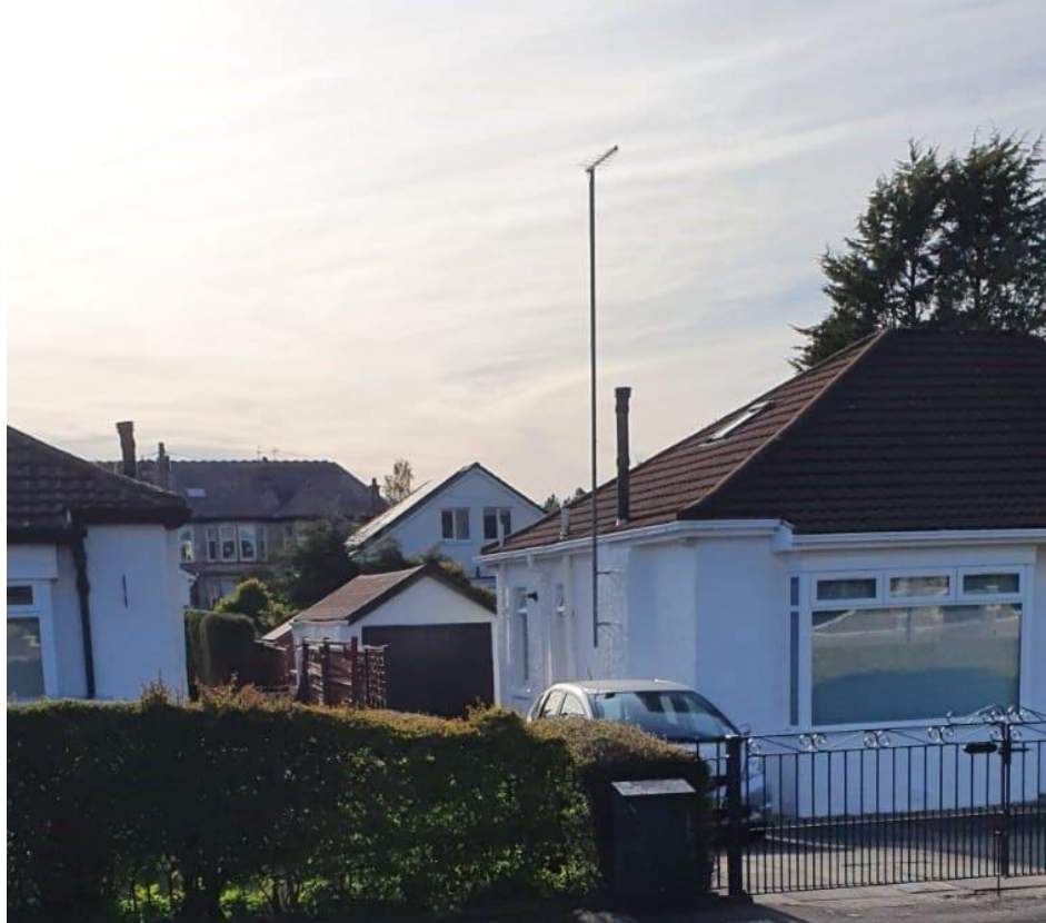
Broomley Drive Gable End Extension taken from Lawrence Avenue
