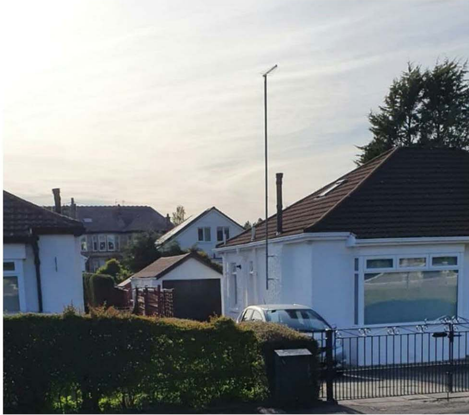
Broomley Drive Gable End Extension taken from Lawrence Avenue
