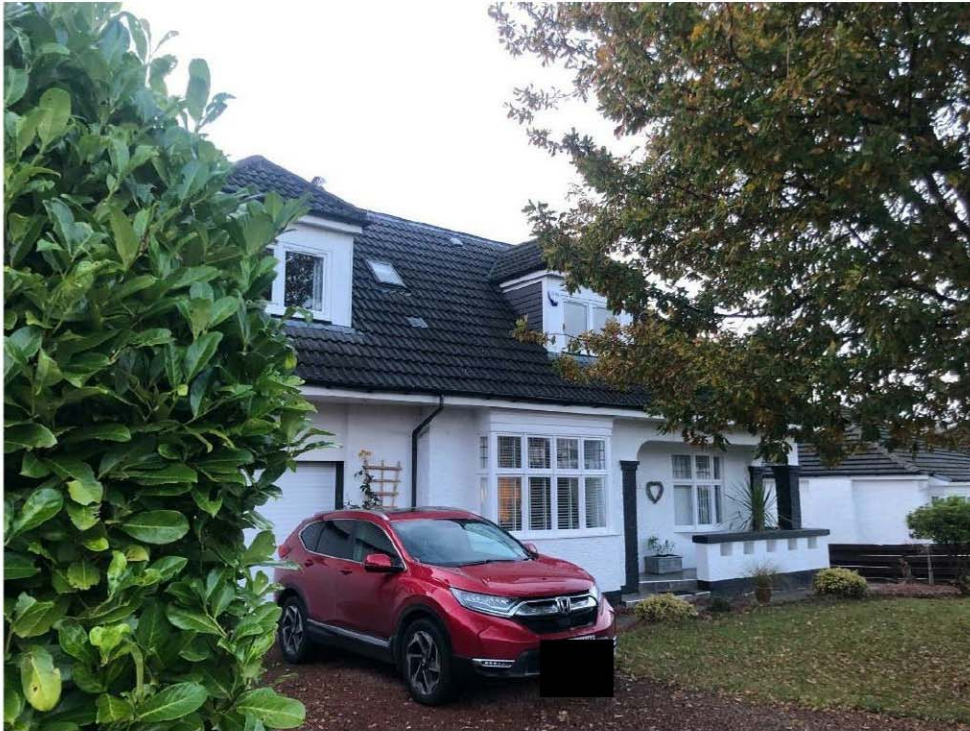
33 Broomley Drive which has been subject to increased roof pitch/height and extension
