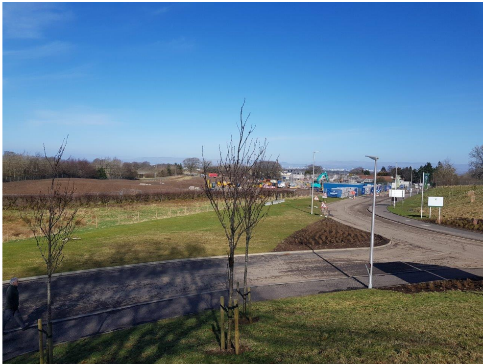
Ayr Rd turns away from application site. Widened grassed verge to East of application site.
