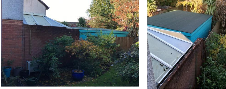
Figure 5: Light impact of neighbouring property- 15 Inverewe Way
