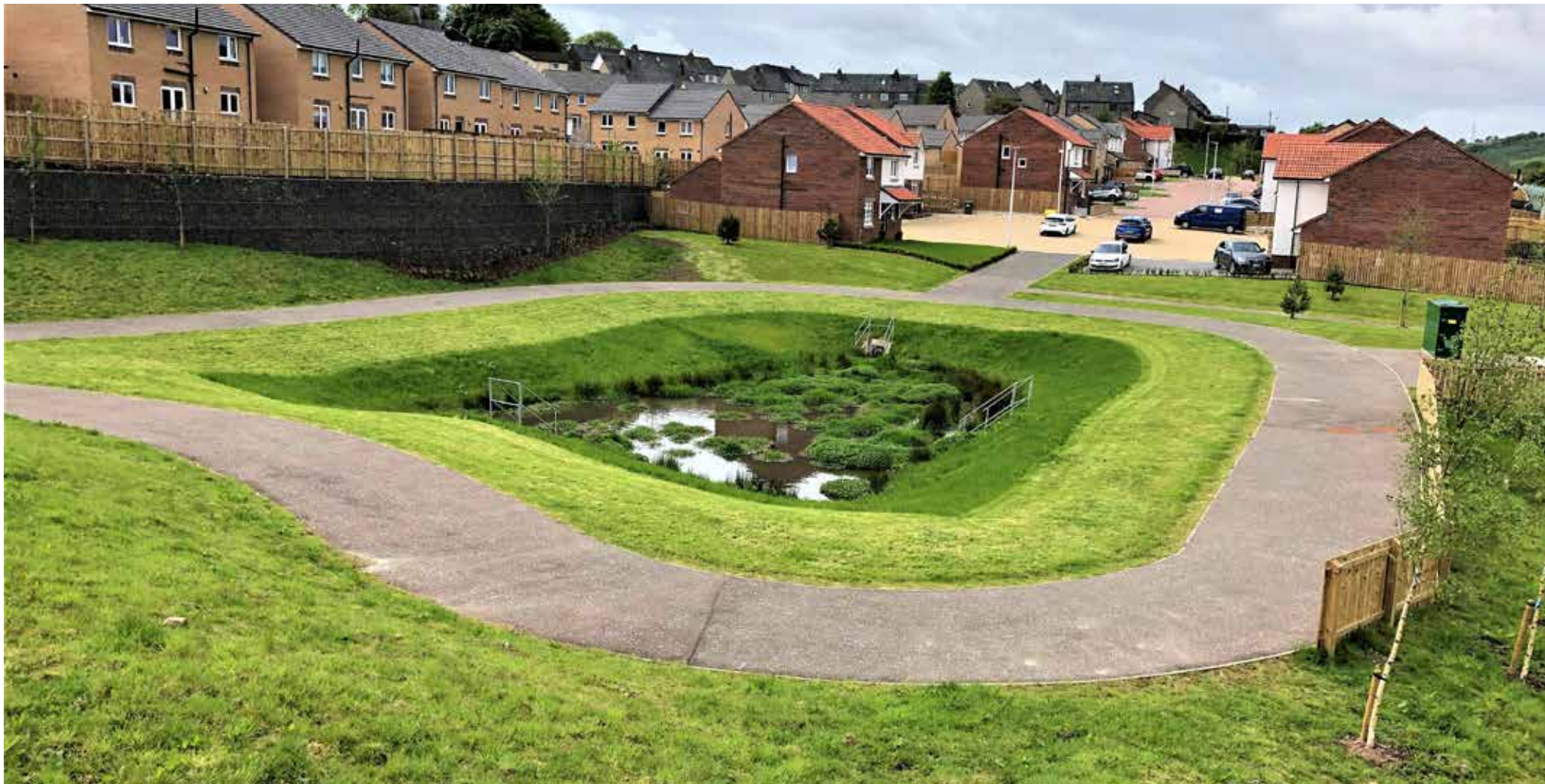
This simple scheme forms the centre point of an accessible area of greenspace.
