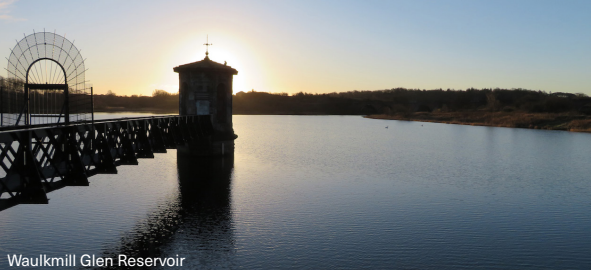
Waulkmill Glen Reservoir
